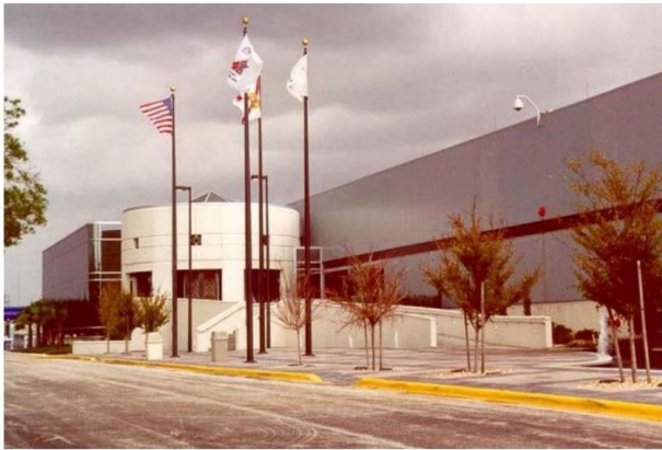
FIGURE 2. AT&T Microelectronics-Lucent Technologies-Cirent agere system front entrance at 9333 South John Young Parkway, Orlando, FL (fab was closed in 2004 and bulldozed in 2010).
