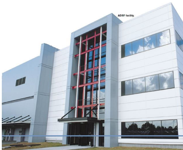
FIGURE 3. Advanced development research facility at 9333 South John Young Parkway, Orlando, FL (fab was closed in 2004 and bulldozed in 2010).
