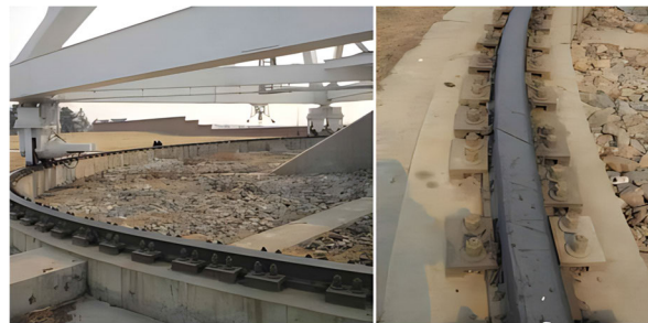
FIGURE 4. Azimuthal track for large wheel-rail antennas. The figure shows the profile of the antenna wheel-rail.
