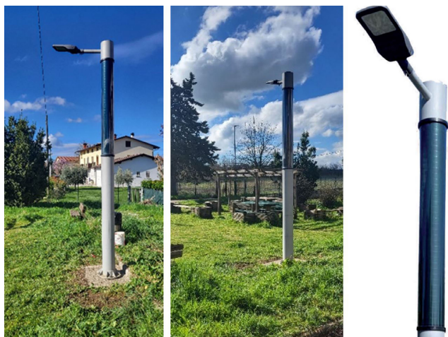
FIGURE 1. Photos of the solar based lamp installed on-site.
