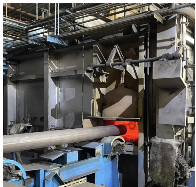
FIGURE 4. Charge side of reheating furnace.
