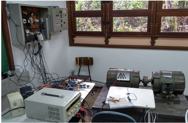
FIGURE 1. Power generation system of small scale of 2 kVA.
