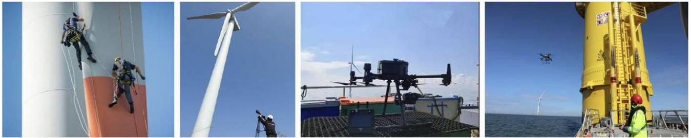
FIGURE 39. Blade inspection utilizing remote and non-remote sensors [146].
