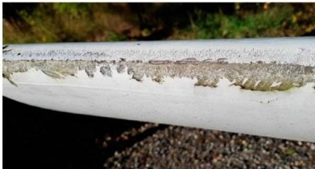
FIGURE 2. Erosion on WTB [6].
