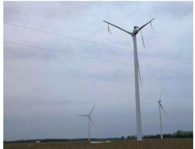
FIGURE 3. Example of a damaged WTB [1].
