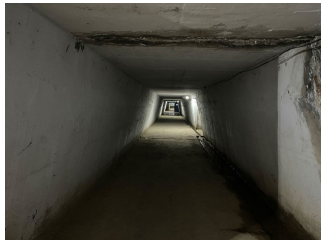
FIGURE 18. Experiment environment in underground tunnel.
