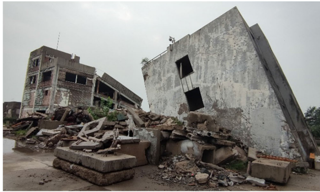
(a) Collapse due to natural disaster
