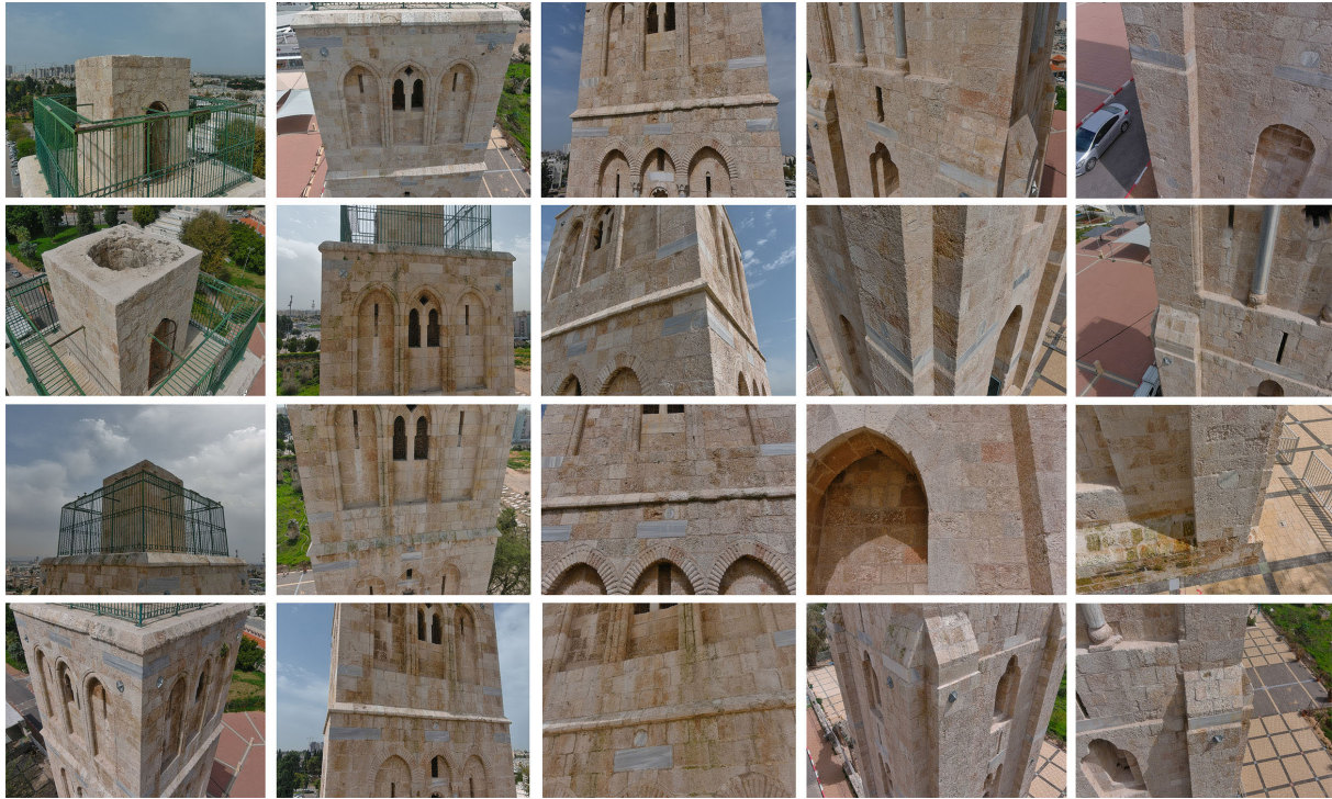
FIGURE 4. A random sample of images captured of the high-rise building by the UAV.
