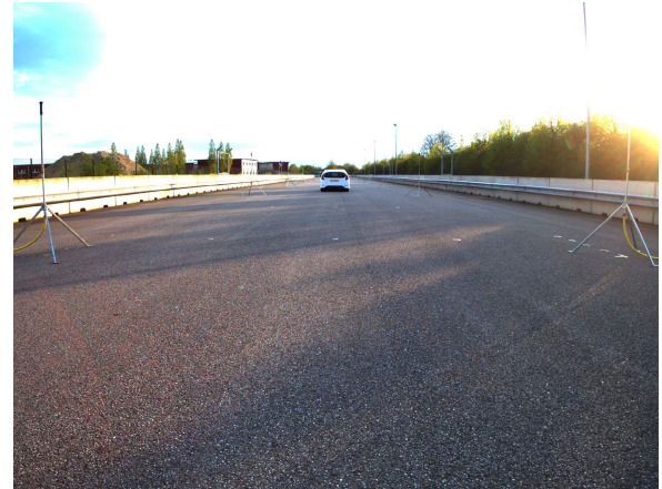
FIGURE 8. Carissima outdoor test facility.
