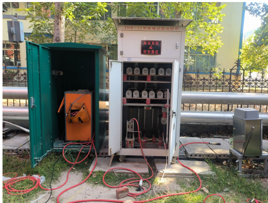
FIGURE 20. On site grounding experimental device.
