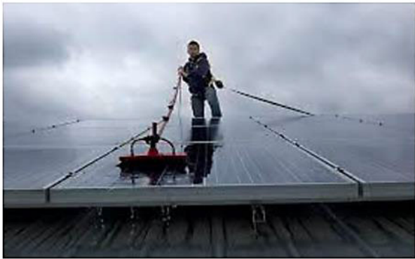
FIGURE 22. Shows the process of cleaning through the utilization of a vacuum section [168].
