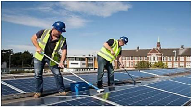
FIGURE 21. Shows a manual cleaning [151].
