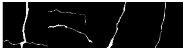
(a) Crack images
