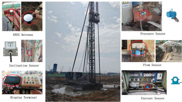
FIGURE 9. On-site installation of high pressure rotary spraying pile sensors.
