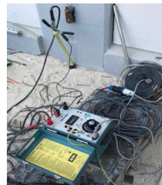
FIGURE 4. DC current test at site.
