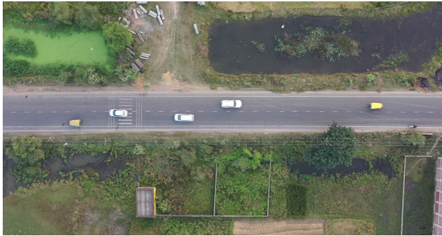
FIGURE 9. Magnified view of the two-lane two-way highway from UAV footage.
