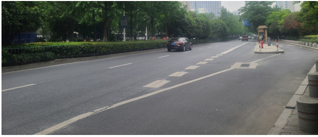
FIGURE 1. A typical bus bay on urban roads in China.
