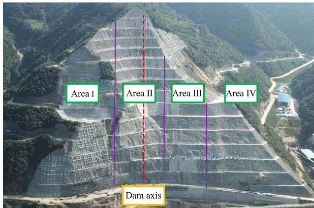
FIGURE 4. Division of left bank slope for a water conservancy project in China.
