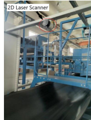
FIGURE 9. The large belt conveyor cycle test system.
