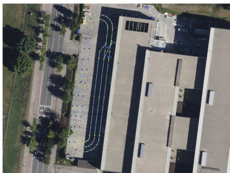
FIGURE 8. Tecnalia Test track.
