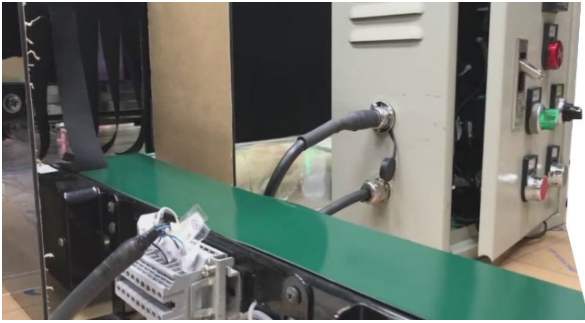
FIGURE 23. The opaque lane controlled by PLC.
