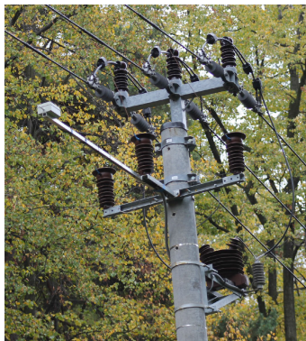
FIGURE 2. Antenna for capturing the signal installed on an overhead power line.
