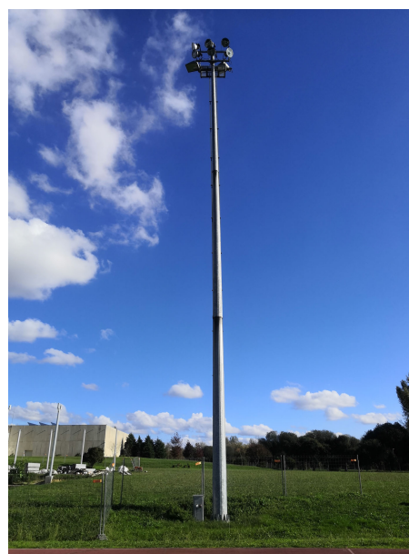
FIGURE 18. Inspected structure: illumination tower of FADEUP's football field.
