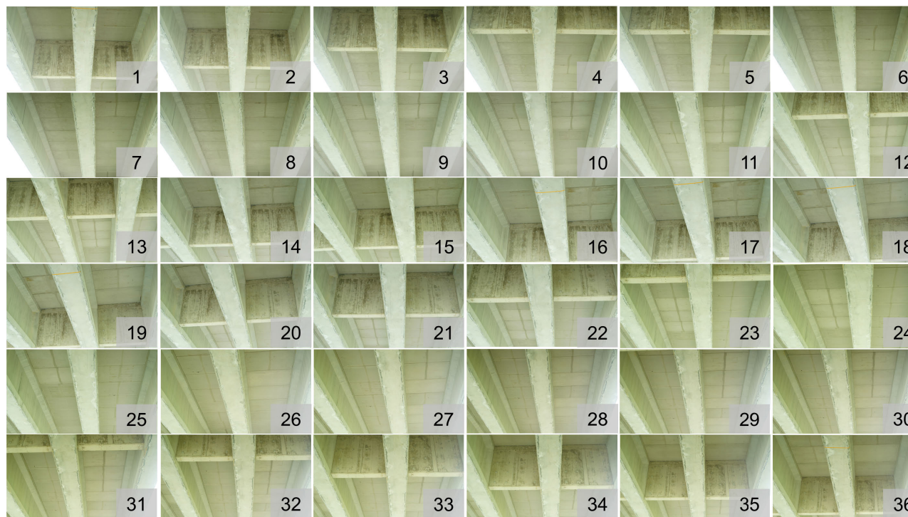
FIGURE 14. Material inspection images for validation 2.
