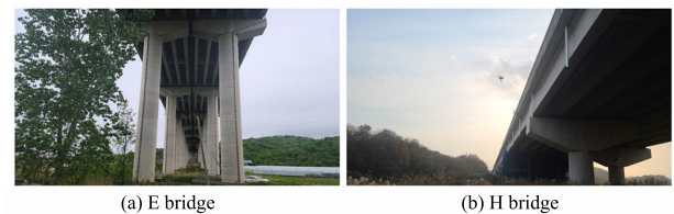
FIGURE 3. Target bridges for inspection image data in stage 1.
