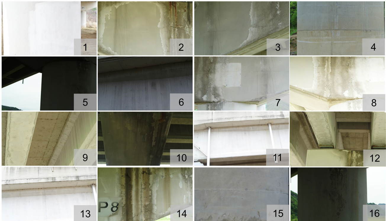
FIGURE 10. Material inspection images for validation 1.
