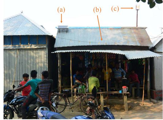
Fig. 18. Swarm microgrid components in operation: (a) SHS installed at a tea stall. (b) swarm microgrid cable connection to neighboring buildings. (c) Telecommunication tower for data connectivity.
