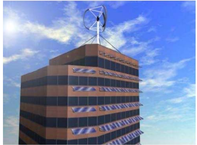
Fig. 2. Wind and PV-based power generation for the vertically integrated microgrid.
