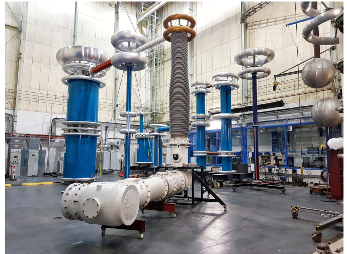
Fig. 4. AC Generator test setup.
