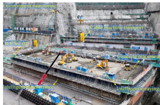
(b) Intelligent technologies used during dam construction
