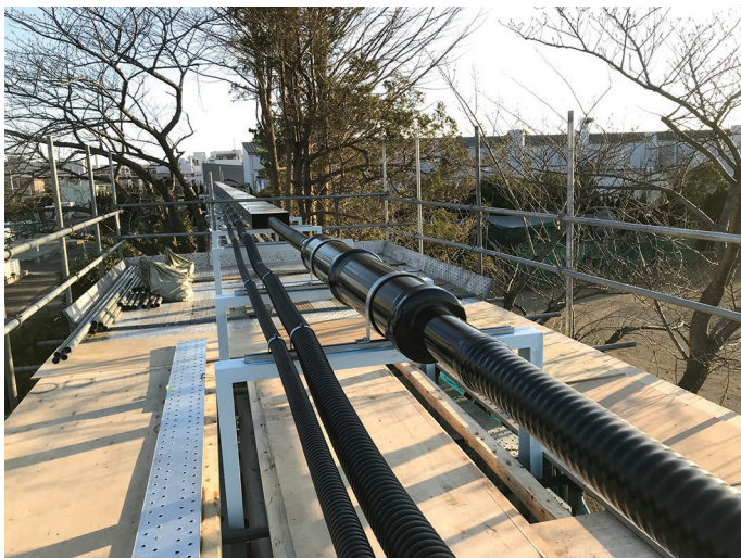
Figure 6. Scene of the verification test, showing the intermediate straight joint.
