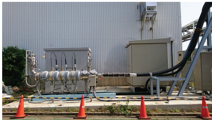
Figure 7. Scene of the verification test, showing the outdoor end termination.
