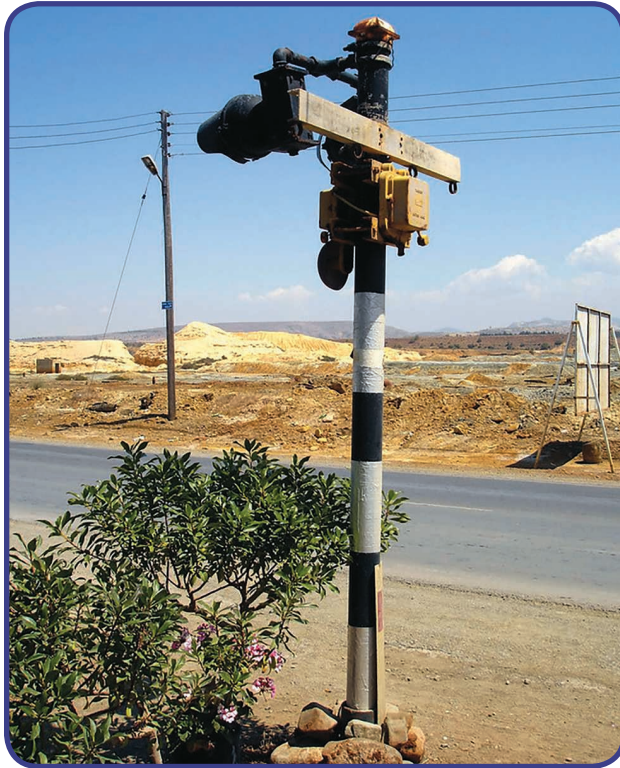
FIG 1 Abandoned railway crossing lights in Cyprus.
