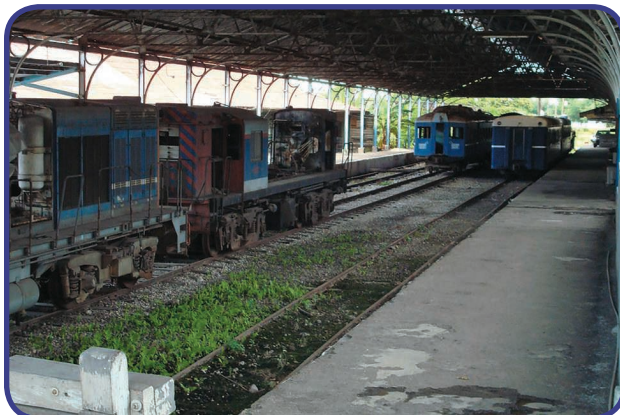
FIG 3 A defunct train station in Jamaica.
