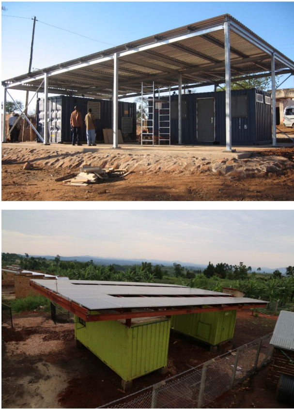
Fig. 4. Top: two-container system under freestanding PV canopy, Kitonyoni, Kenya. Bottom: two containers integrated into the canopy system, Kyamugarura, Uganda (no water collection).
