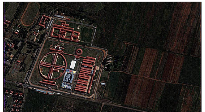
Fig. 23. Example of monitoring of Zondervoort Correctional Center [120].
