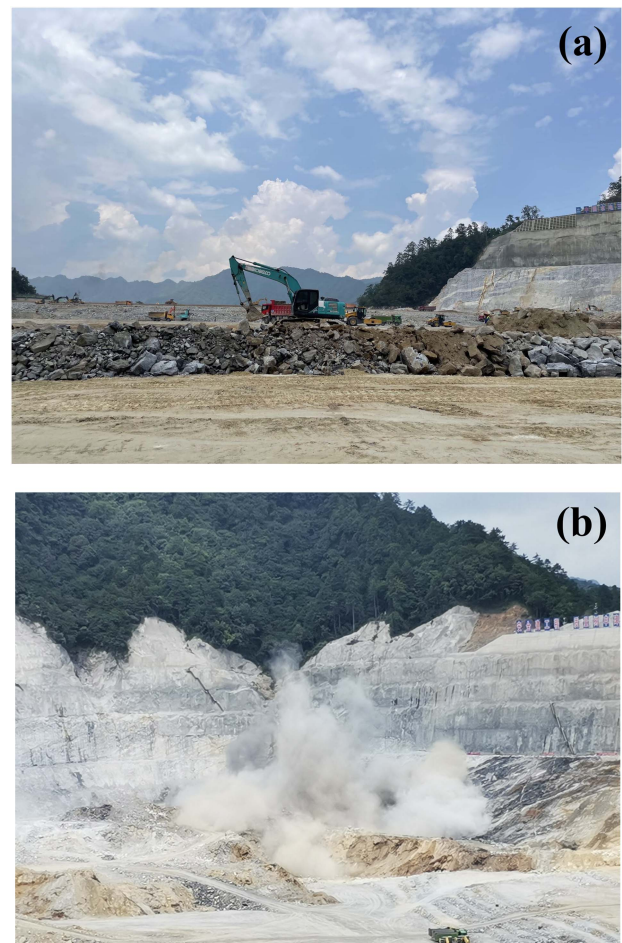
Fig. 13 (a) Site construction photography. (b) Blasting remote view.
