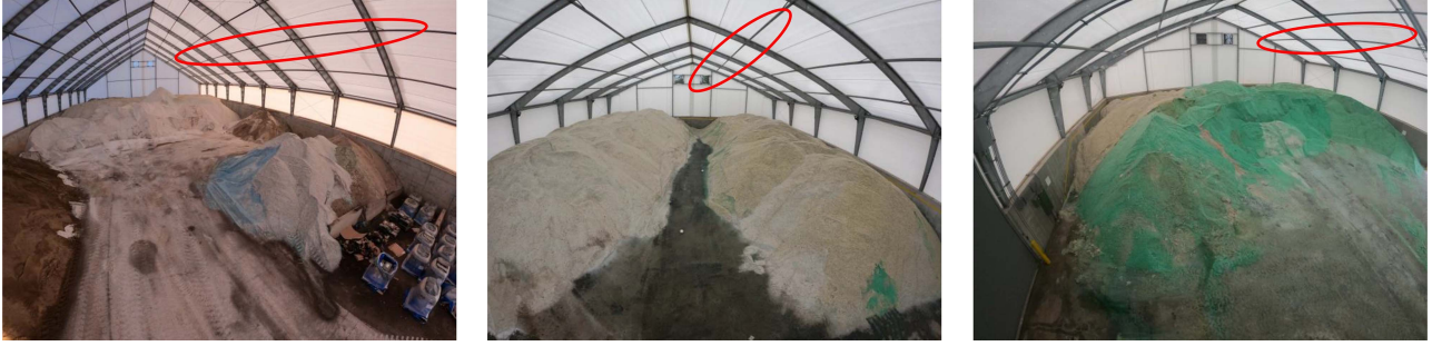
Fig. 10. Illustration of sample linear features in indoor facilities highlighted with red ellipses where the majority of line segments are located near planar features.
