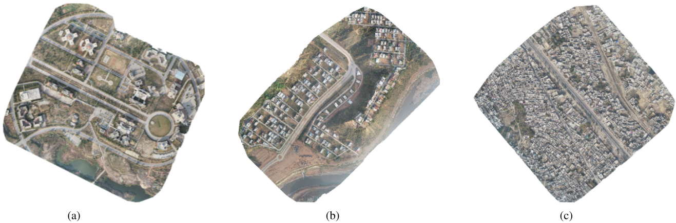
Fig. 5. Geo-tagged Orthomosaics of three different areas. (a) A geographical patch from NUST Islamabad which covers about 0.522 \text{ km}^2 area. (b) Area in DHA Rawalpindi having sparsely populated terrain and covering upto 0.64 \text{ km}^2 area. (c) Densely populated urban area of Gujar Khan District in Pakistan which represents 0.664 \text{ km}^2 land. (a) NUST. (b) DHA. (c) Gujar Khan.
