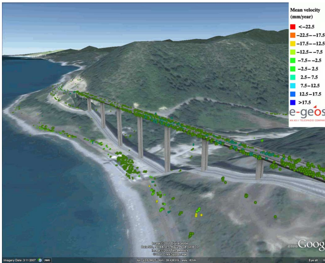
Fig. 5. Viaduct of the Sochi–Tuapse highway, Russia. 3-D view showing accurate positioning of PSP mean velocity measurements obtained from COSMO-SkyMed SAR data (35 descending Stripmap SAR acquisitions, February 2009–December 2010).
