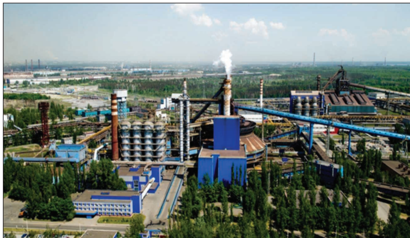
FIGURE 12 – The Novolipetsk Steel facility in Lipetsk, Russia.
