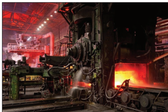
FIGURE 10 – A rolling mill machine.
