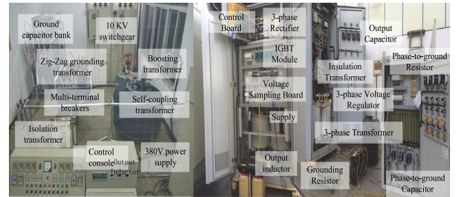
Fig. 14. Experimental platform for flexible grounding system of distribution network.
