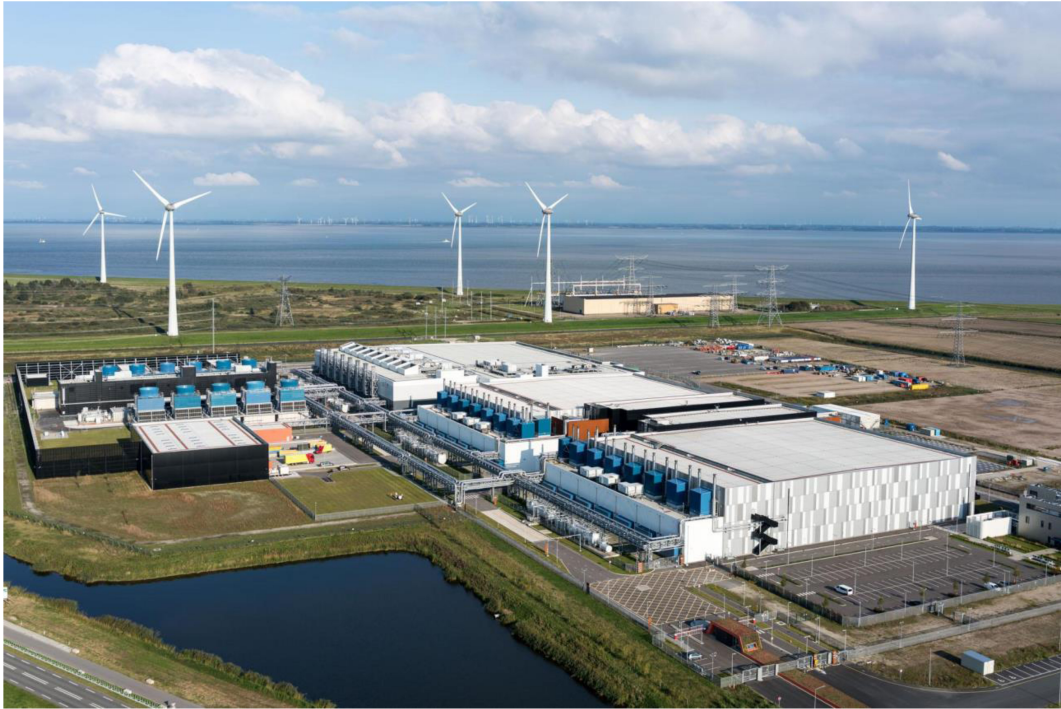
FIGURE 1. A Google warehouse-scale computer in Belgium.
