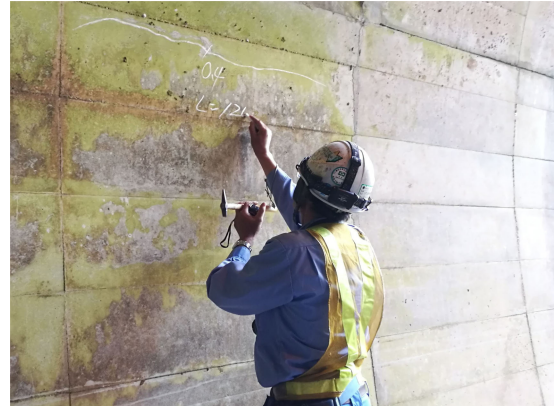
Fig. 1. Hammering test being conducted in a tunnel.
