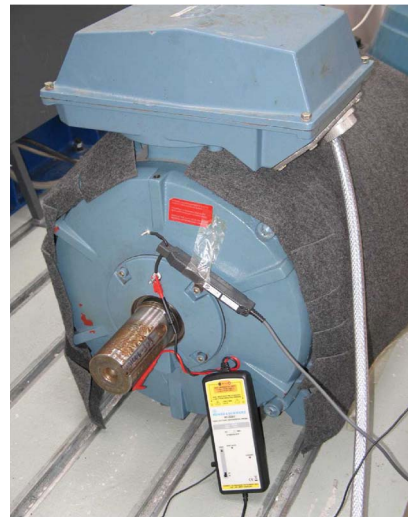
Fig. 3. Measurement setup of motor MB-75 (75 kW).
