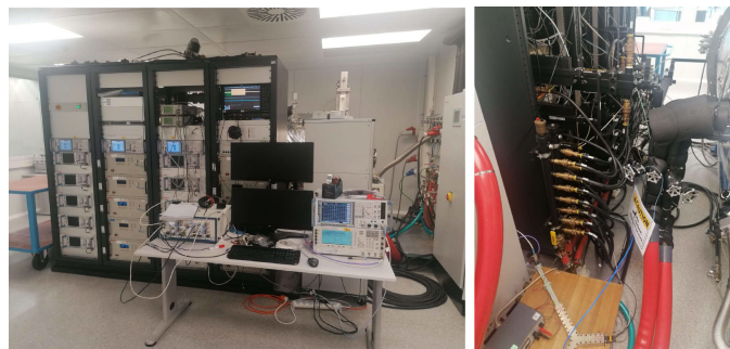
Fig. 3. Assembled PIM setup based on the multicarrier facility for the first set of PIM measurements.
