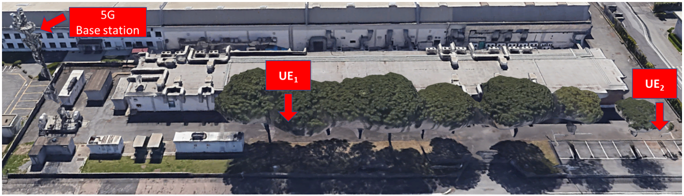
Fig. 4. Measurement site and UE position.
