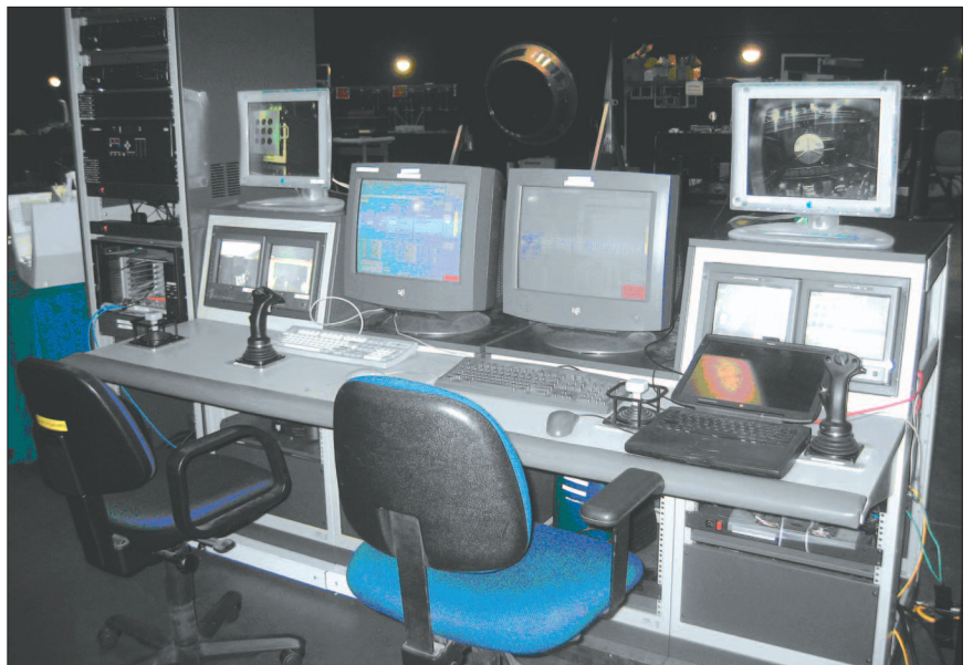
Figure 2. Typical Ranger control station configuration.
