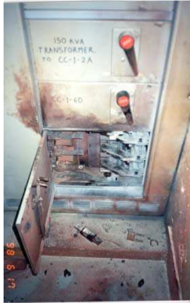
Figure 48—Low-voltage class circuit isolation equipment (top view) where Peter Wiebe was engulfed in the discharge of the arc-flash products (heat, spatter, plasma)
