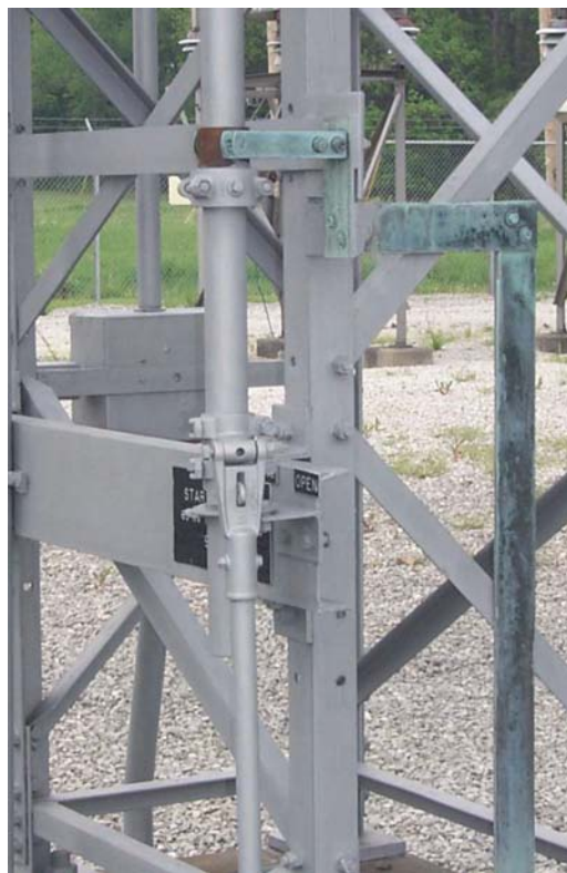
Figure 36—Typical braidless grounding device
