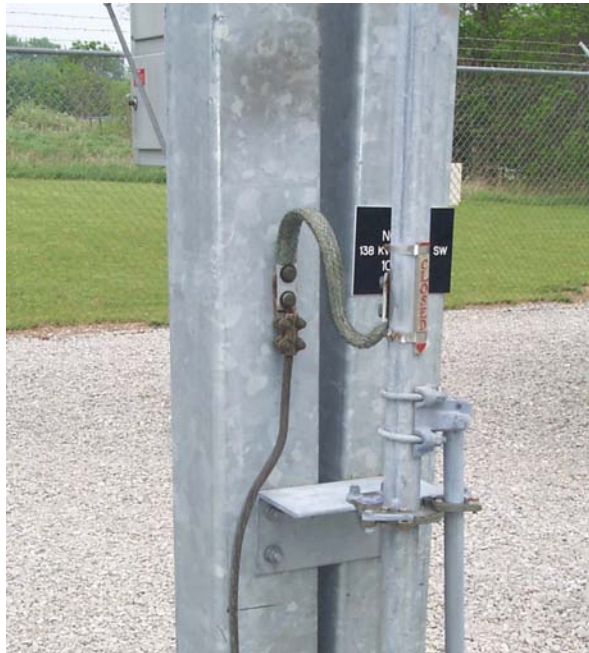
Figure 35—Typical braided ground
