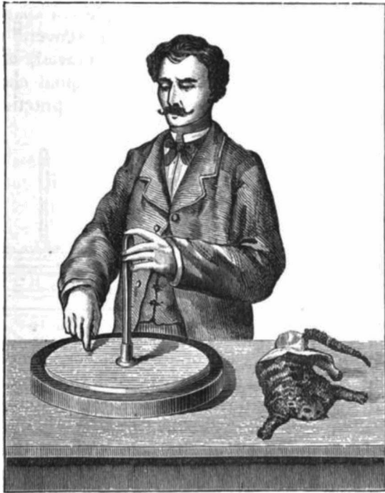
Fig. 26. Drawing showing the operation of an Electrophorus, a simple manual electrostatic generator invented in 1762 by Swedish Professor Johan Carl Wilcke. Image by Amédée Guillemin (died 1893).
