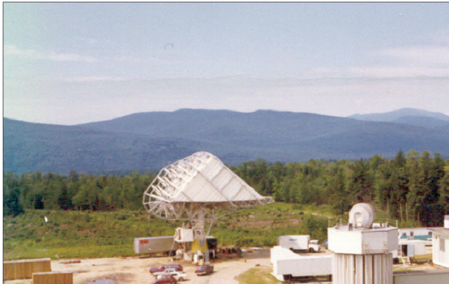
Figure 3. The AT&T designed 30-m Andover, Maine Earth station as photographed in 1966 (courtesy of Comsat Legacy Project).
